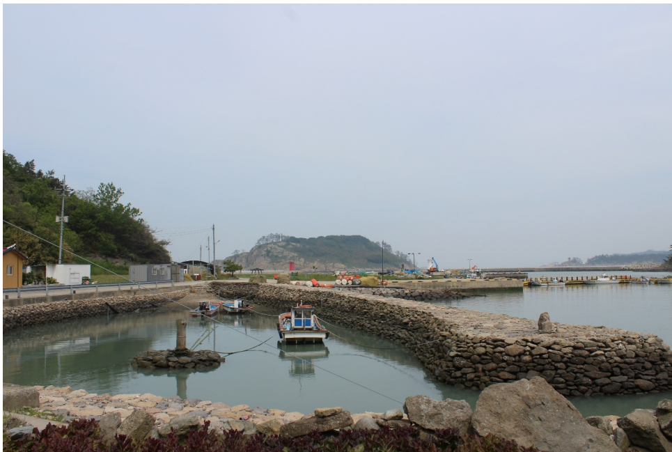
Fig 1. Traditional use of natural resource materials for harbor (photo credit: Samantha Chisolm Hatfield)
